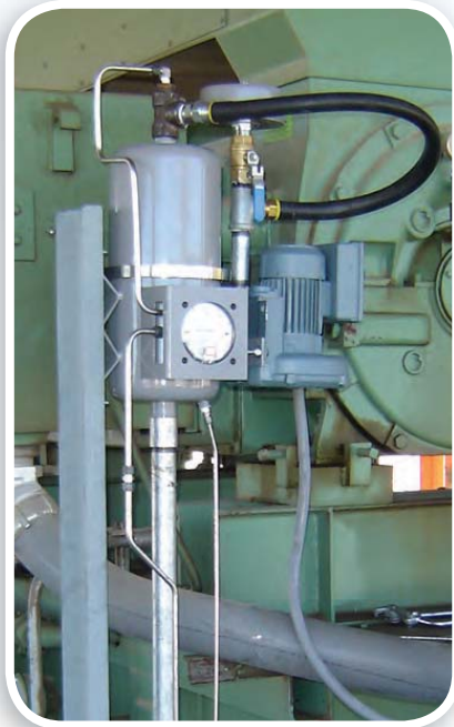
Cooper TA11000 Compressor Vacuum Assisted Oil Mist Eliminator
