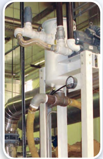
Caterpillar G3520 Engine/Gen-Set Landfill Gas to Energy Application Vacuum Assisted Oil Mist Eliminator
