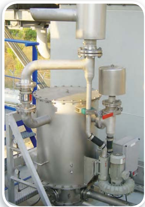
GE LM2500 Gas Turbine Stainless Steel Vacuum Assisted Oil Mist Eliminator.
